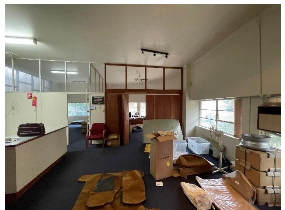
First floor mezzanine level offices to be demolished.
