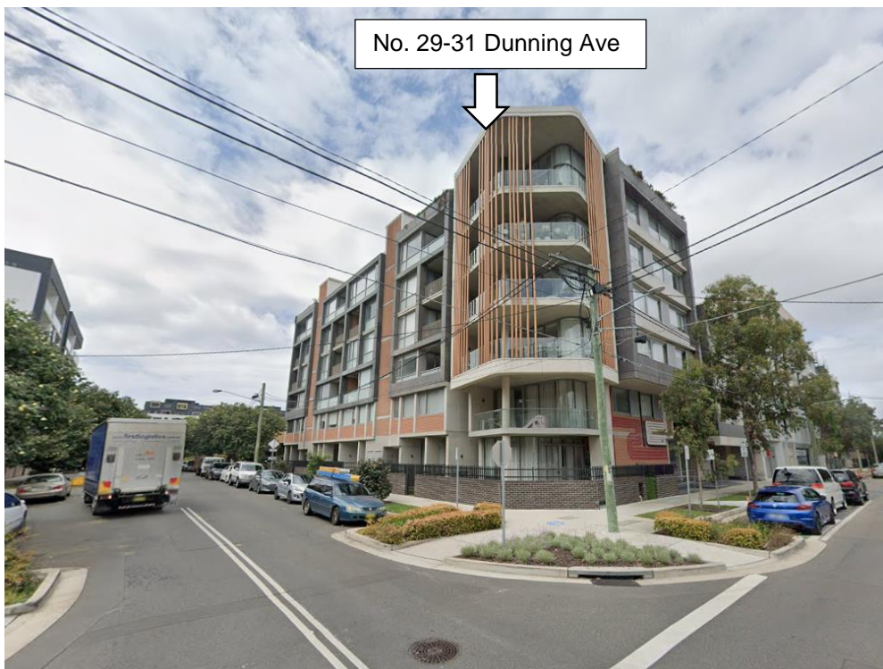
Figure 7: Number 29-31 Dunning Avenue, residential development to the south of the subject site
