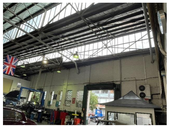
Existing openings and vertical steel columns which are proposed to be removed and altered.
