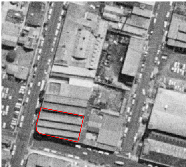
Figure 21: Aerial of view of site circa 1950 showing the saw-tooth roof and completed warehouse
